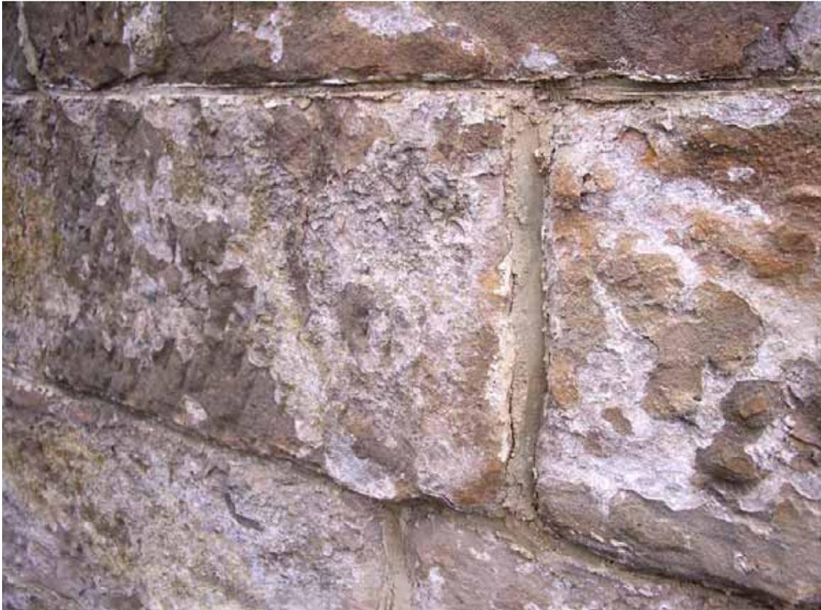
Figure 8 – Efflorescence of salt forming on the face of the stone of the gaol walls, with some flaking beginning to occur. Note that the pointing was replaced in 2003.
