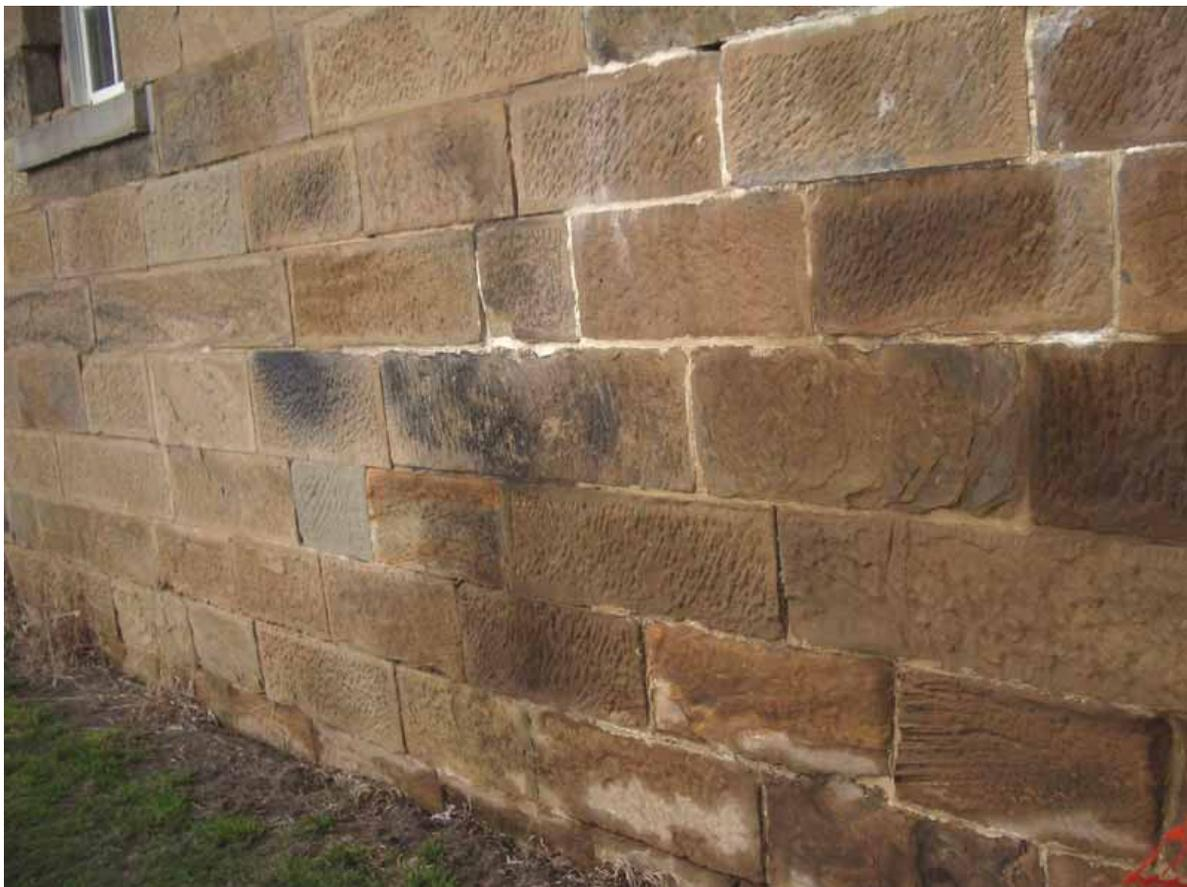
Figure 6 – The dark areas on the gaol walls are distinct patches of moisture. The ground level inside the walls is at the fourth course shown here.
