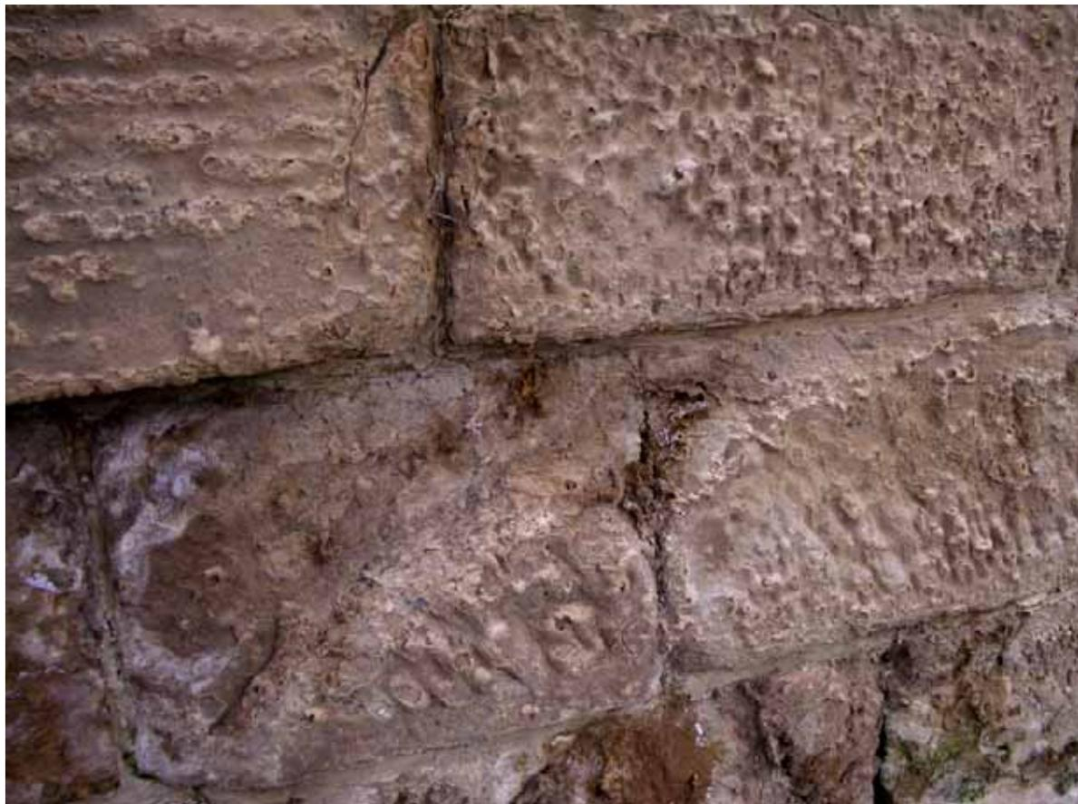
Figure 9 – Severe flaking and blistering of the face of ashlar blocks.
