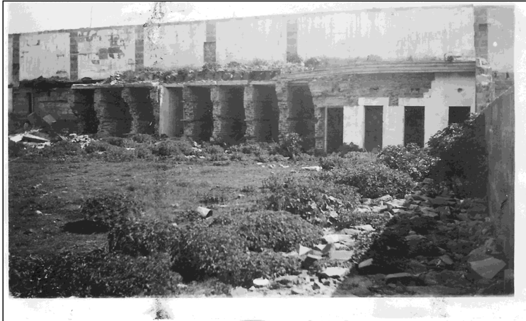
Figure 6.5 – Demolition of the Men’s Division, late 1937 – the area of excavation will cover the two right-most cells. Photograph: Oatlands District Historical Society.
