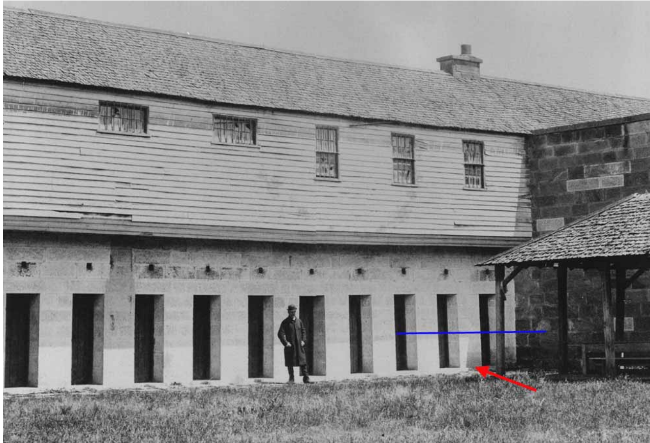
Figure 6.4 – The Men’s Division solitary cells c1910 – the area of denoted by red arrow, the blue line denoting likely current ground level. Photograph: State Library of Tasmania.
