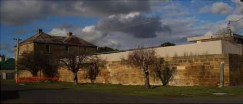
Figure 1.4 - Northern wall of the Oatlands Gaol – the Gaoler's Residence (left) and pool fence/buildings (right).
