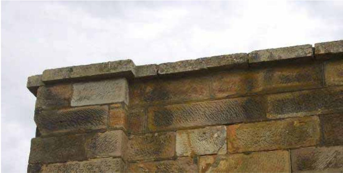
Figure 172 – Capstones on top of the relocated gaol arch, High Street, Oatlands. These are likely to be original capstones from the gaol walls.
