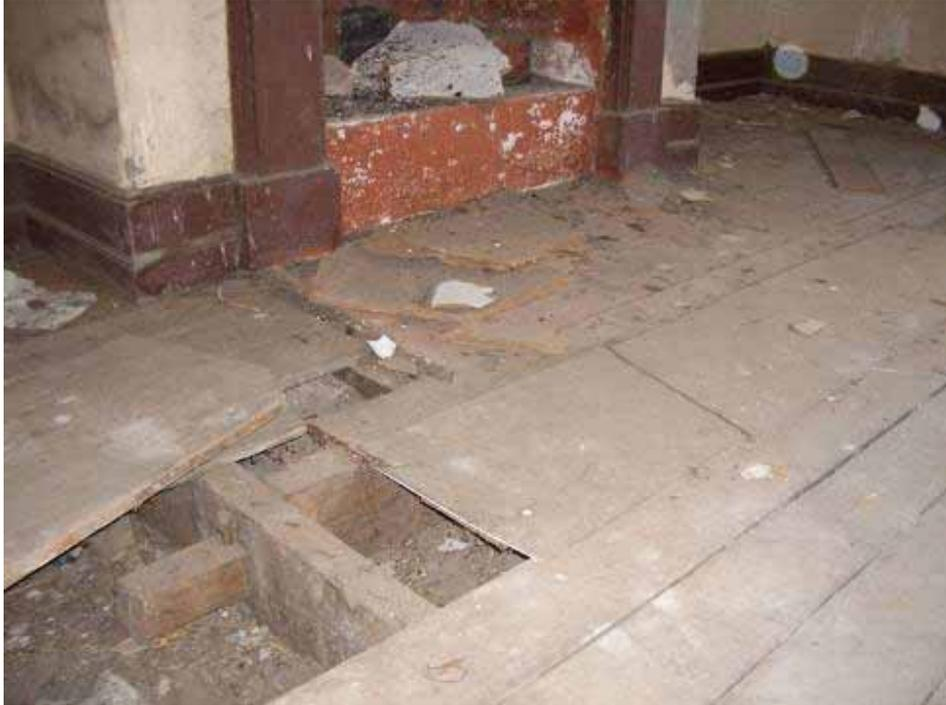
Figure 153 – Substantial floor framing of the upper level of the Gaoler's Residence, showing pegged and morticed joints.
