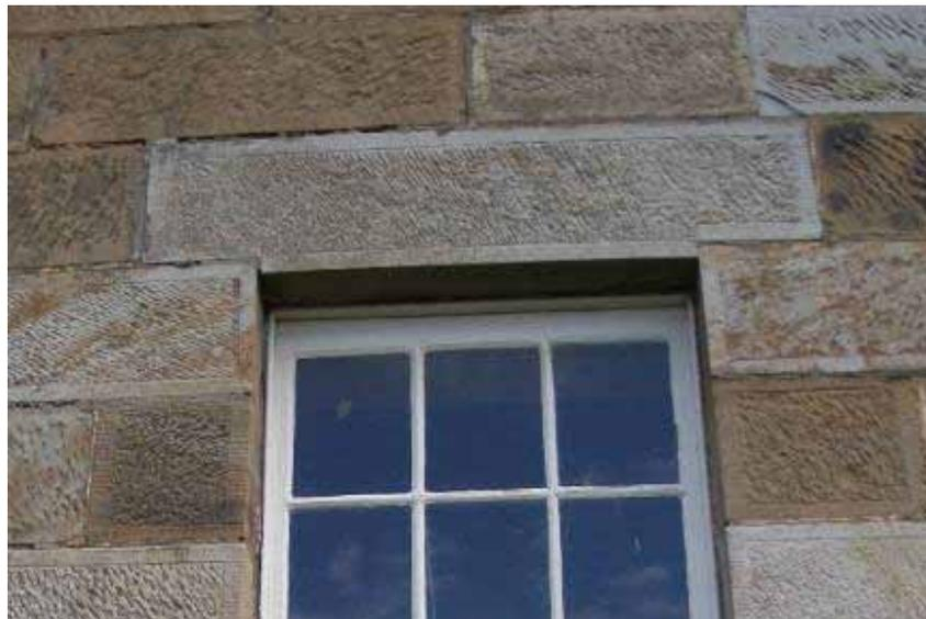
Figure 166 – The subtly more articulated lintel style of the Gaoler's Residence showing a shaped base rather than being a squared block spanning the opening. This style represents about half the lintels in the building.
