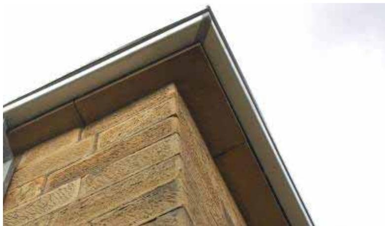
Figure 159 – Sandstone capstones which form the eaves of the Gaoler's Residence.
