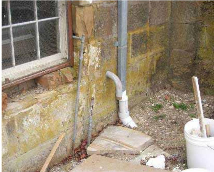
Figure 170 – An example of the various externally-run services entering the Gaoler's Residence.
