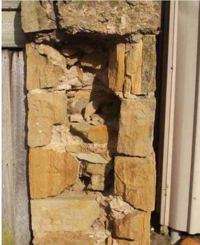
Figure 161 – Internal rubble/mortar fill of walls, as seen on demolition scar to the east of the original main gates site.
