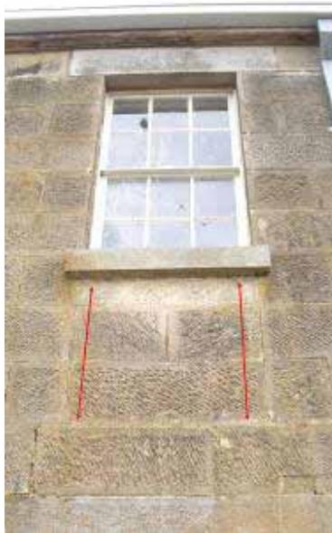
Figure 131 – Red lines indicating vertical joints running the height of 3 courses of stone between the window of the former parlour, possibly indicating a former doorway.
