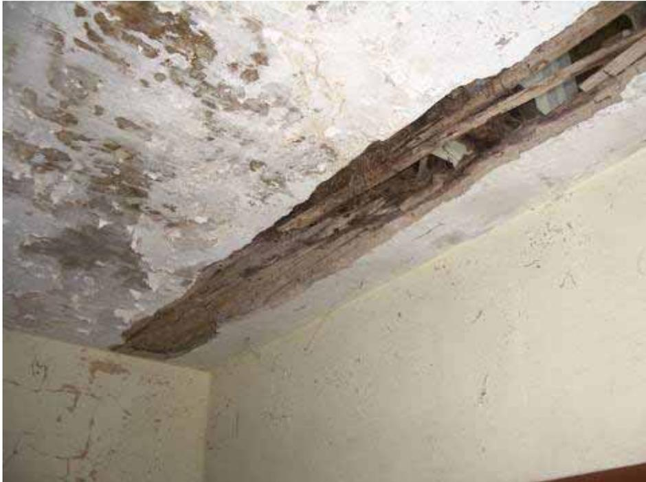
Figure 88 – Failing ceiling in 1.1, the result of an inadequate valley gutter.
