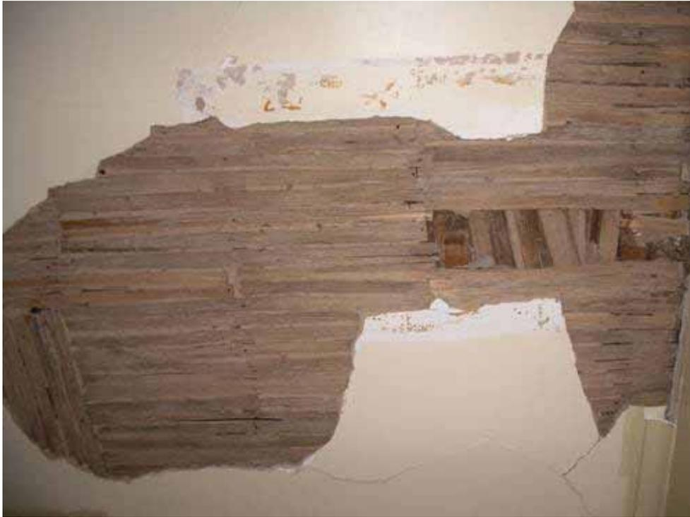
Figure 125 – Section of collapsed ceiling in G6, showing the split lathe beneath. Note also the modern cornice.
