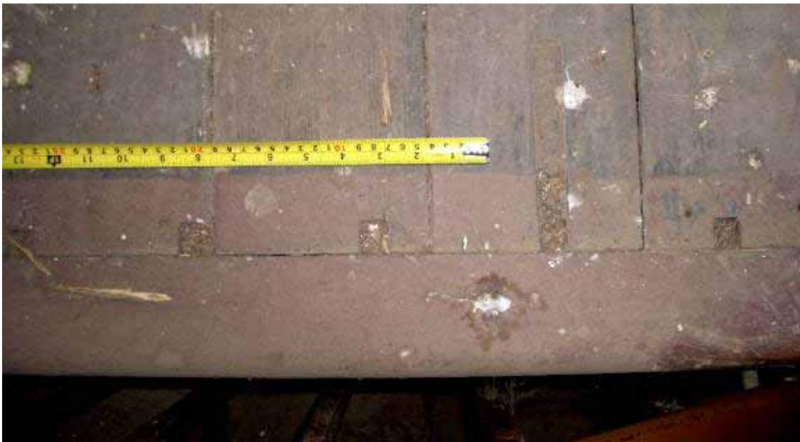
Figure 148 – Part of a brass balustrade support, and line of rebates to house uprights in the floor of 1.3.
