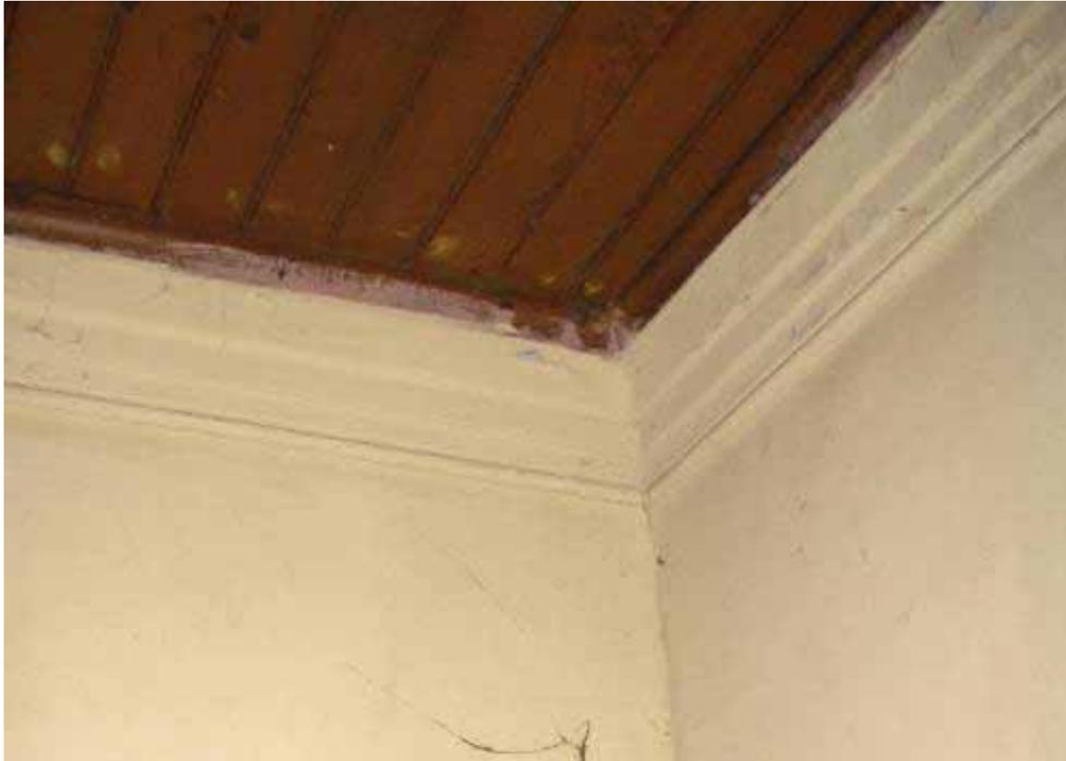
Figure 114 – Baltic pine ceiling and plaster cornice in G4.
