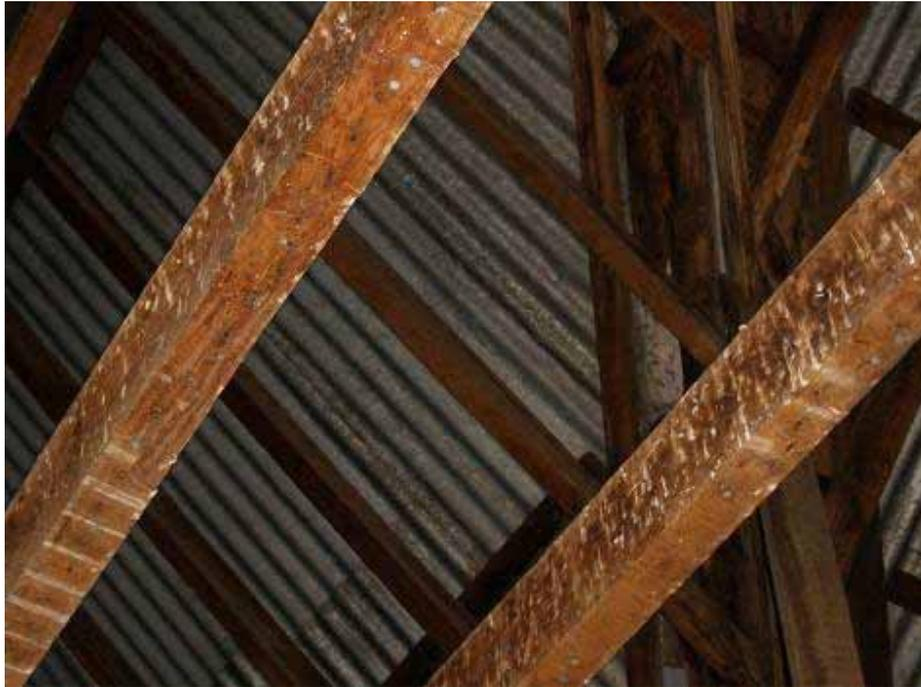
Figure 157 – Roofspace above the Gaoler's bedroom (1.4). Note the evidence of the former lathe and plaster ceiling.
