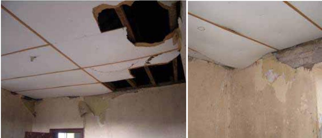
Figures 154 (left) and 155 (right) – Collapse of the Caenite ceiling in the former Gaoler's Bedroom (1.4).
