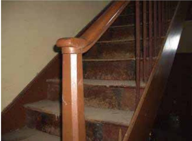
Figures 115-118 – Detail of the stairs, showing the original white sandstone steps beneath the newer pine casing, also the profile of the banister railing.
