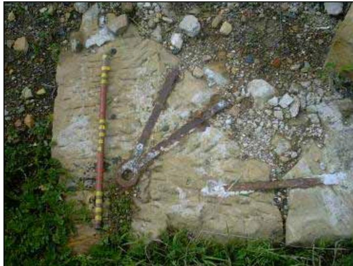
Figure 176 – Iron hinge-pin rebates, installed with lead plugs, remaining on the original foundations of the gaol arch at the Oatlands Gaol.
