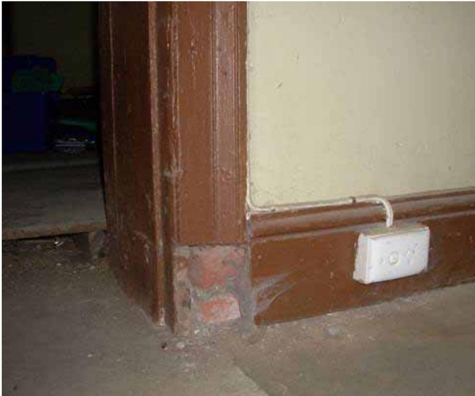
Figure 127 – Bottom of doorway between G6 and G5 showing internal brick wall, and architrave shortened to accommodate a raised floor previously removed from that room.
