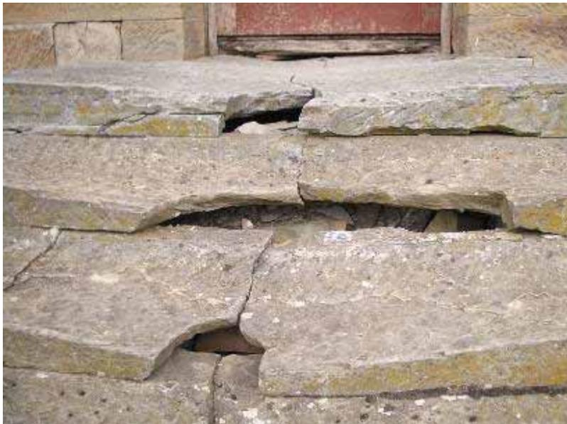
Figure 168 – Rubble fill, probably quarry tailings, beneath the steps leading to the Gaoler's Residence – see also Williams (2003:105).
