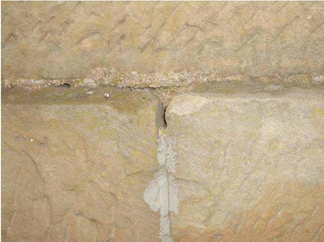
Figure 163 – Examples of pointing on the façade of the Oatlands Gaoler's Residence, showing a very early lime-based mortar (horizontal) and a more recent (and inappropriate) cement based mortar (vertical).
