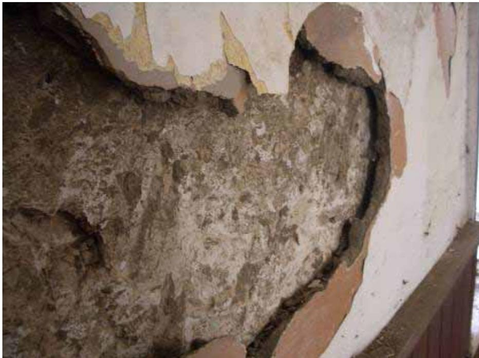
Figure 103 – Detail of the paint and plaster layering in the former Women's Kitchen (G3). Note the painted surface beneath the plaster, which indicates that the room once had painted stone walls. See also Figure 79.
