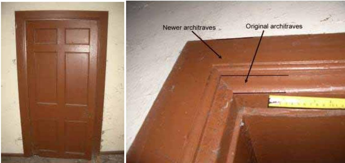
Figure 90 (left) – 6-panel door between G1 and G5 – a typical style throughout the building. Figure 91 (right) – The two layers of architraves in G2 demonstrate an attempt to redecorate that room.
