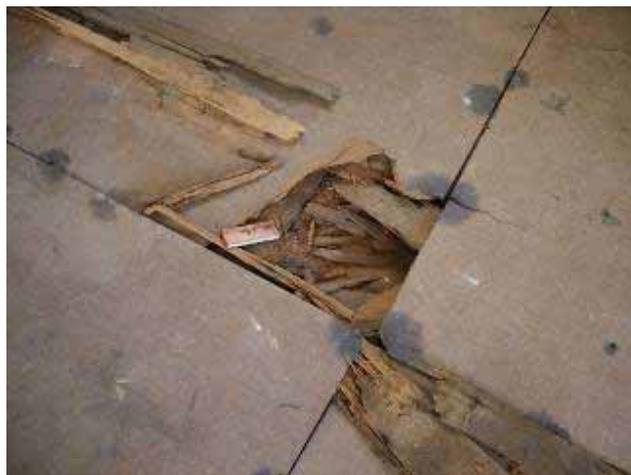
Figure 96 – Rotten floorboards, seen through Masonite in G3. The original flagstones can be seen through the rotten timber.
