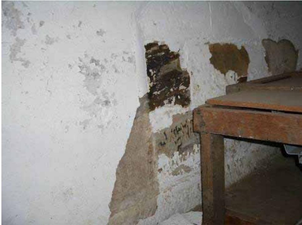
Figure 79 – Detail of plaster and surface finishes, southern wall of G1. This shows remnants of early paint beneath the more recent plaster, as also observed in G3 (see Figure 103)..
