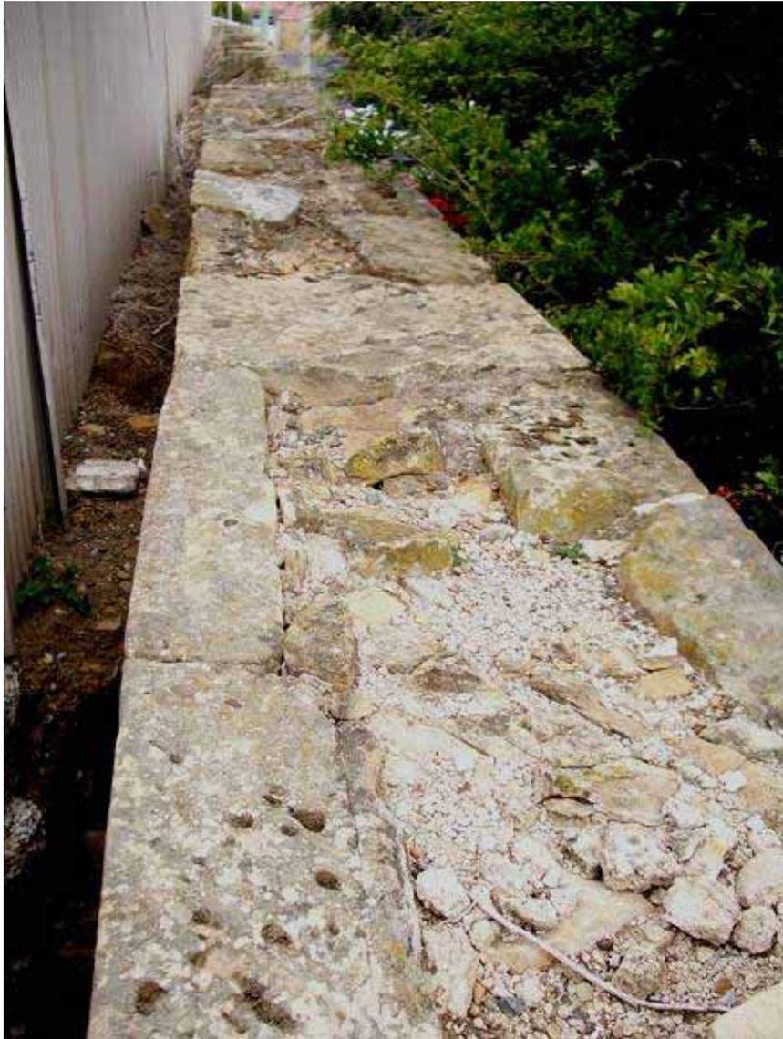
Figure 171 – A typical portion of the current top of the gaol walls, the incomplete demolition leaving the rubble/mortar inner fill exposed.
