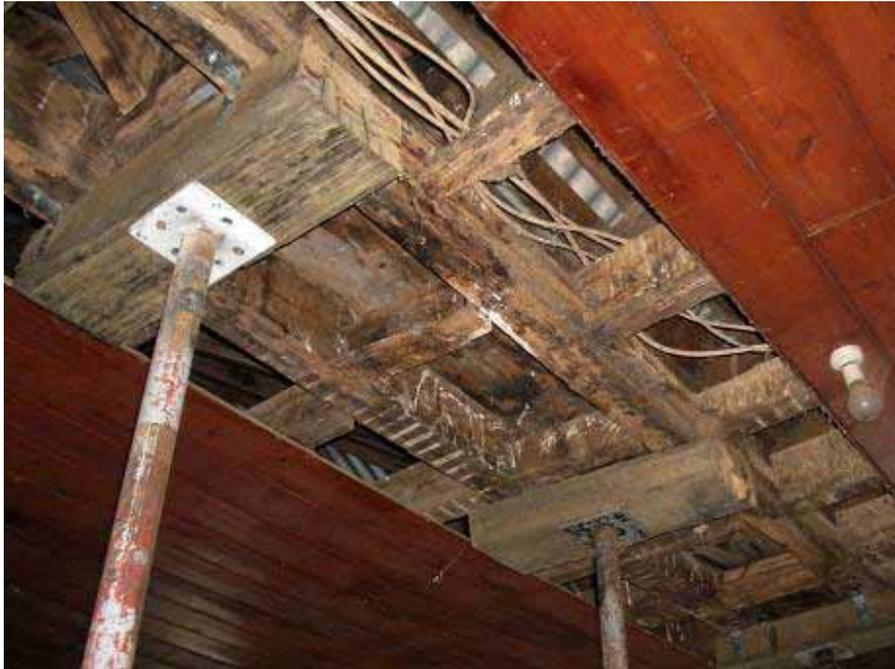
Figure 134 – Baltic pine lining on the ceiling of 1.1. Roof structure can be seen, supported by temporary props to prevent imminent collapse.
