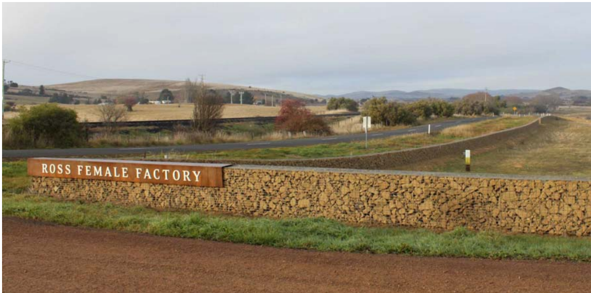
Figure 8 – Examples of gabion walling at an historic site, Ross Female Factory (installed 2009).
