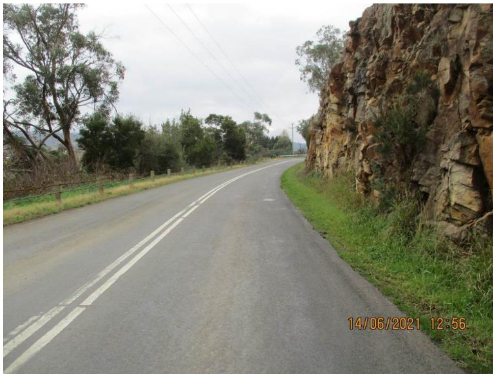
Photograph 4: View to east along Elderslie Road from rear of vehicle turning right into Black Brush Road
