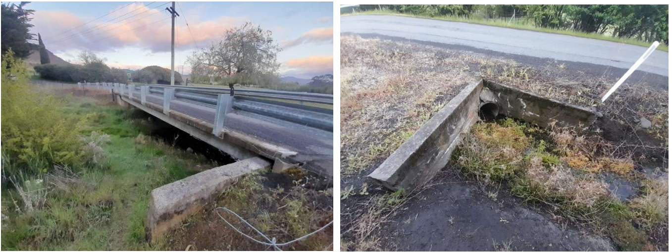
Figure 10. (L) Sugarloaf Road bridge (R) Culvert under Sugarloaf Road
