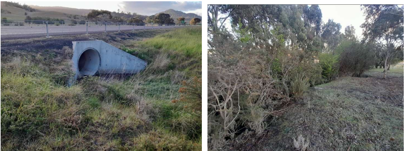
Figure 8. (L) Discharge culvert beneath Midland Highway (R) Overgrown Glenfern Creek
