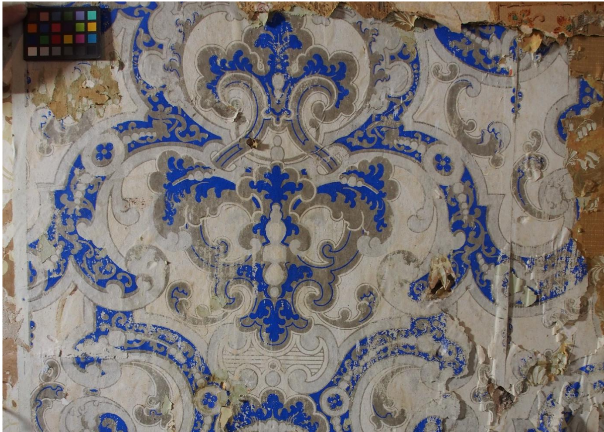
Figure 1: Wallpaper ca 1855 discovered in the Judges Chamber (layer 2 of 18), Oatlands Supreme Court House. This wallpaper was chosen to provide a suitable grandeur for the Judge's Room, achieved through the use of brilliant blue which had, until the early 1850s, been far too expensive for wallpaper.
