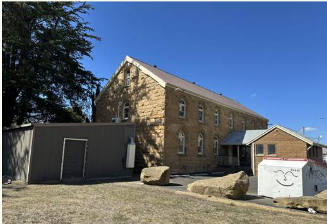
1 Heritage Campania Flour Mill building with recent building additions of varying materials
