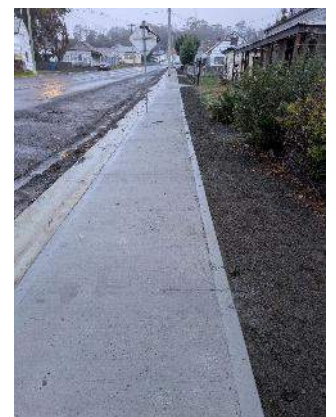
Parattah kerb replacement
