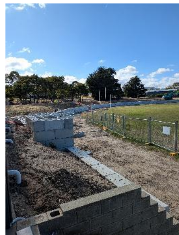
Campania Football Club retaining wall works
