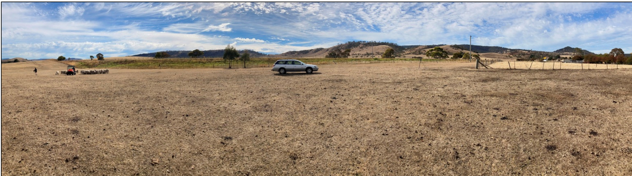
Eastern panorama of highway boundary from near Location 1, 19/3/2026
