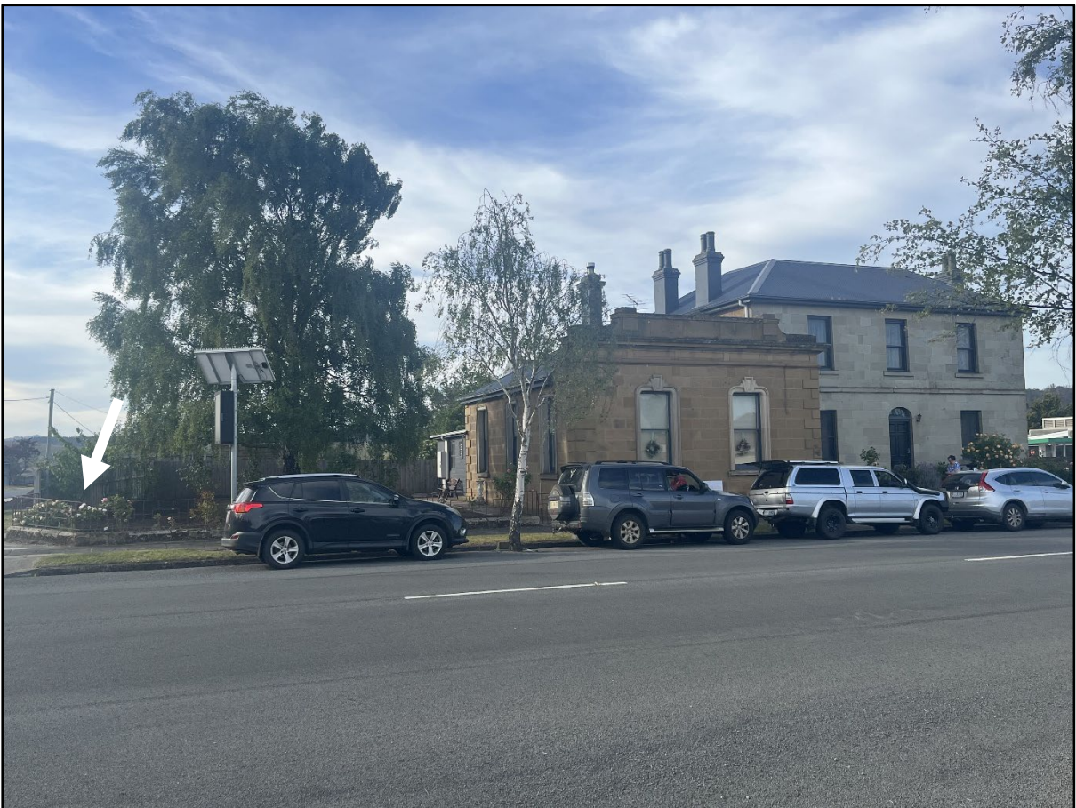
FIGURE 1. SITE AS VIEWED FROM HIGH STREET WITH SIGN LOCATION SHOWN
