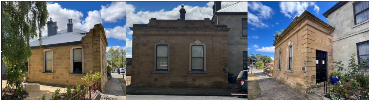
FIGURE 9. THREE PRINCIPAL ELEVATIONS OF THE FORMER ANZ BANK. THE SIGN WILL NOT IMPEDE ANY OF THESE VIEWS.
