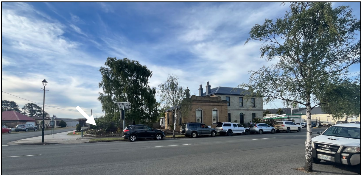
FIGURE 12. VIEW OF THE SITE FROM HIGH STREET WITH SIGN LOCATION NOTED.
