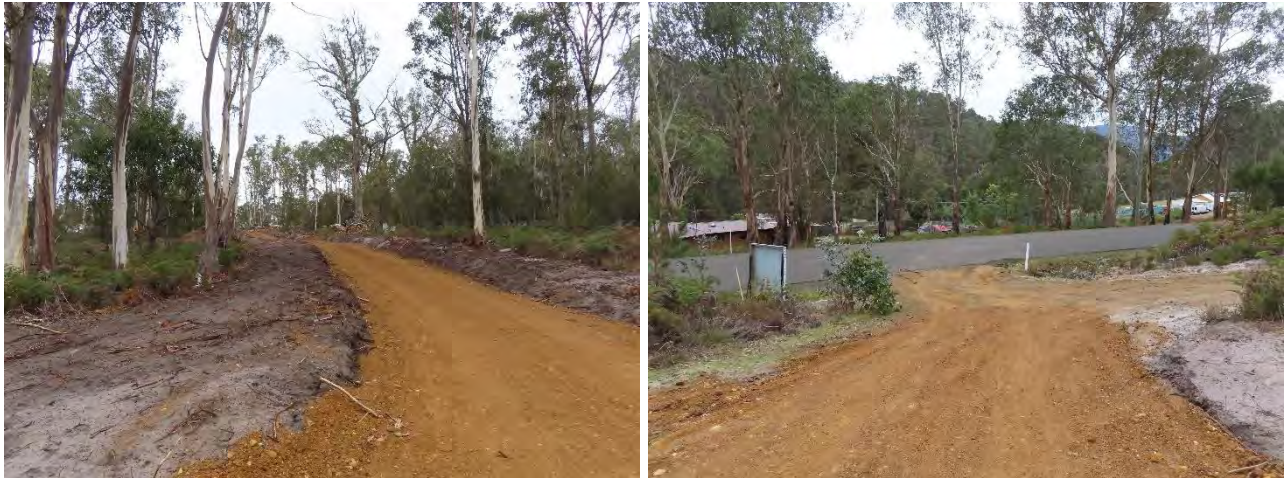
Plates 1 & 2. Views of the existing well-formed access
