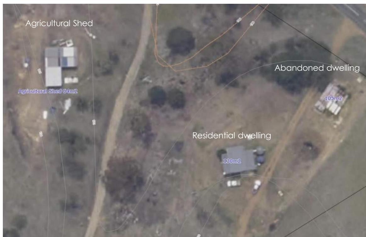
Figure 6: Aerial image showing the buildings on the Property.
