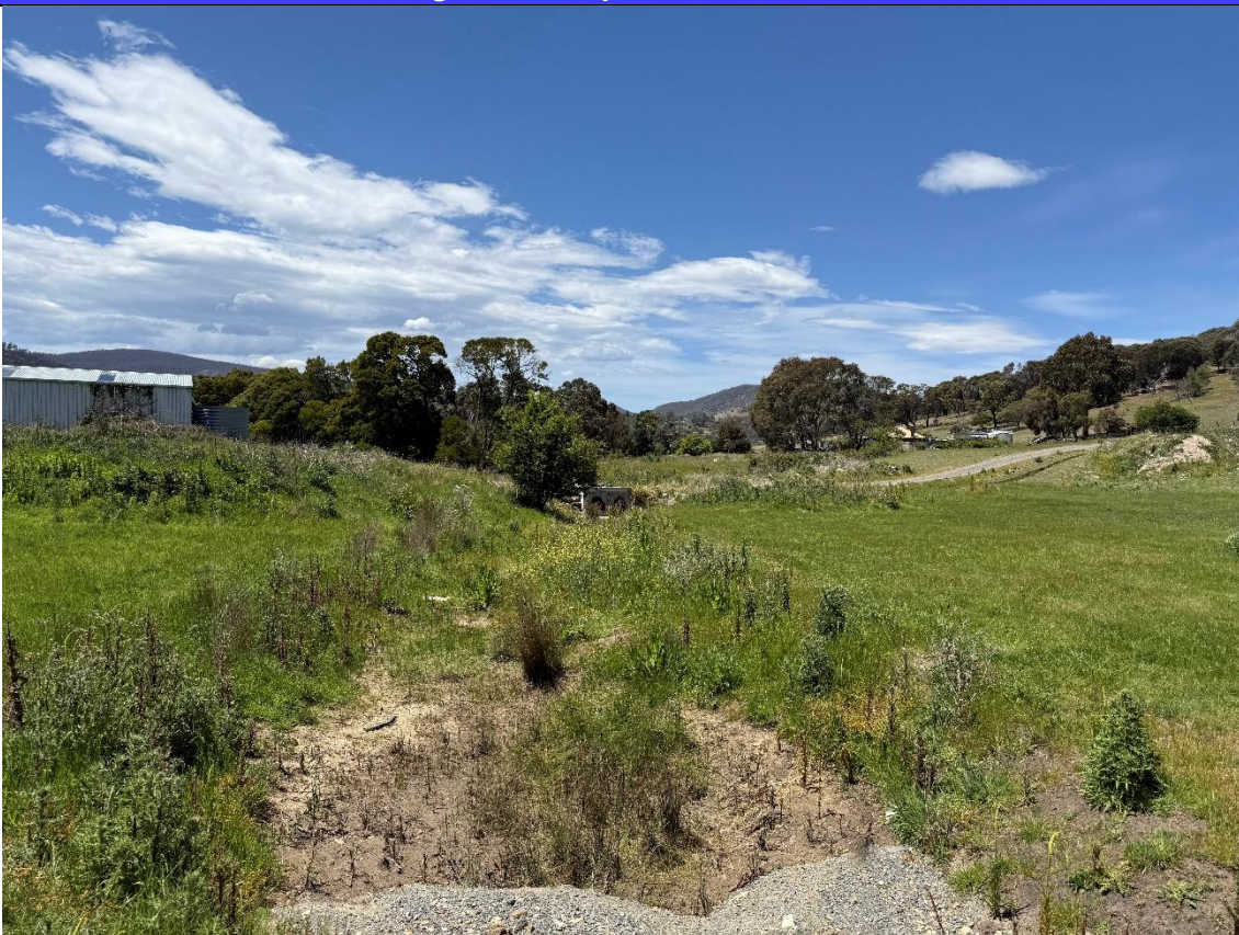
Image 4: Downstream of outlet
