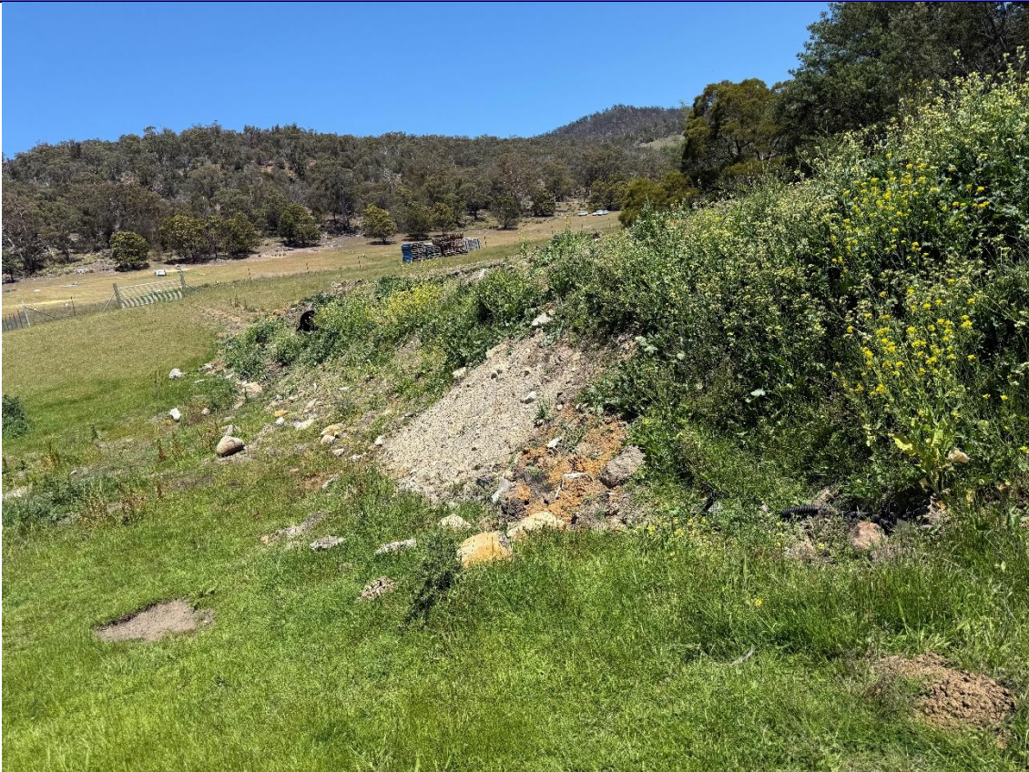
Image 3: Partially Stabilised Batters
