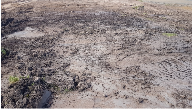
Figure 1 - Stripping of subgrade organics
