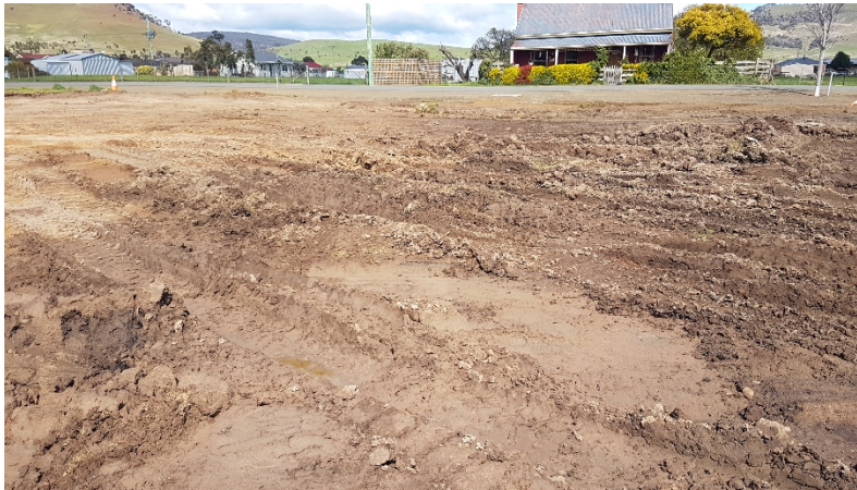
Figure 2 - Subgrade stripping with 'soft spots'
