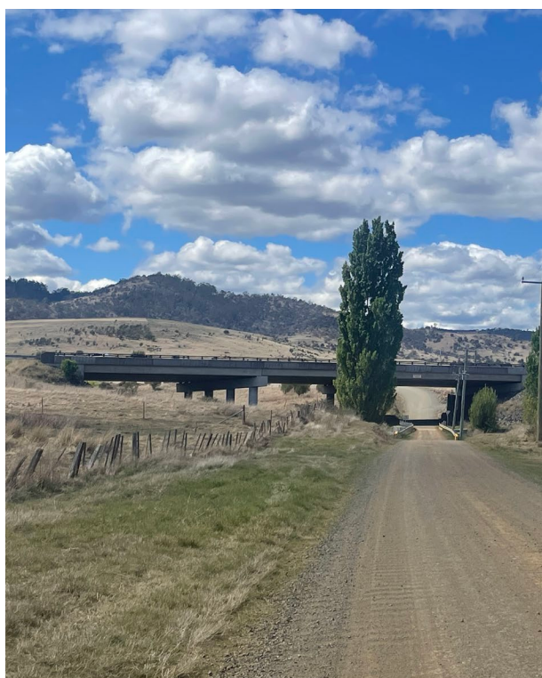
Figure 12 – Subject site southern frontage
