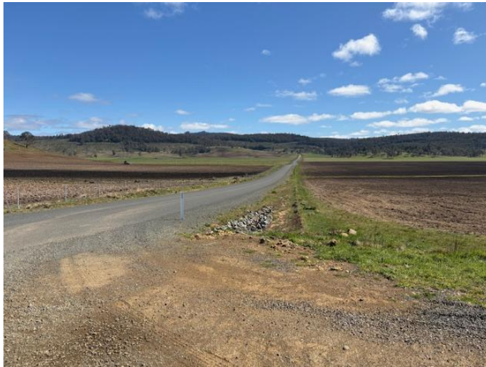
Figure 22– Looking right along Interlaken Road from farm access
