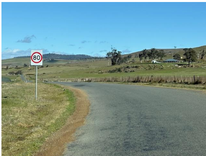
Figure 7 – Looking West along Interlaken Road from Oatlands
