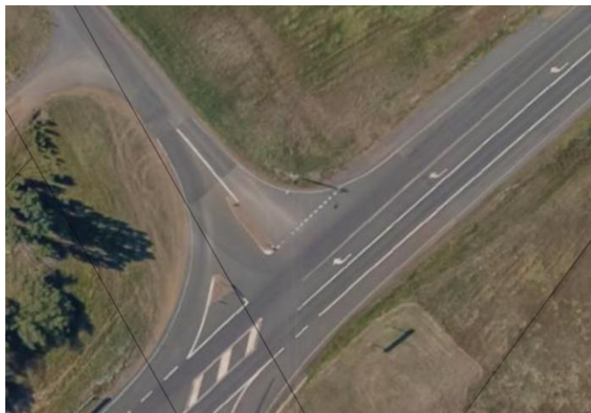
Figure 10 – Aerial view of Midland Hwy/ Interlaken Rd junction
