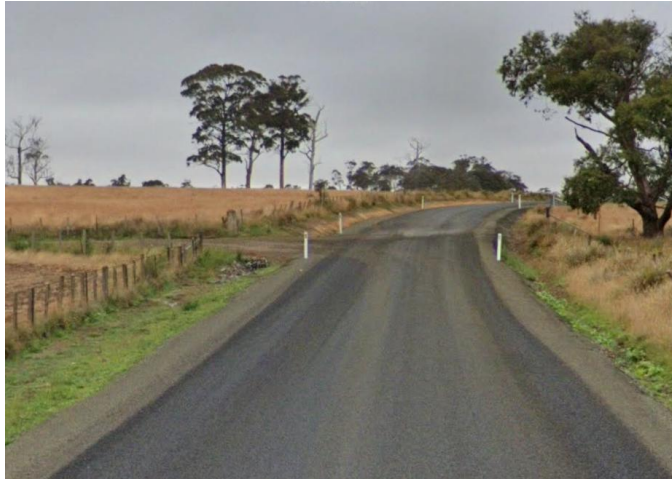
Figure 25 – Interlaken Road Western approach to farm access
