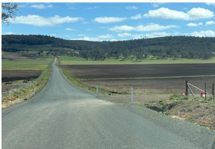
Figure 24 – Interlaken Road Eastern approach to farm access
