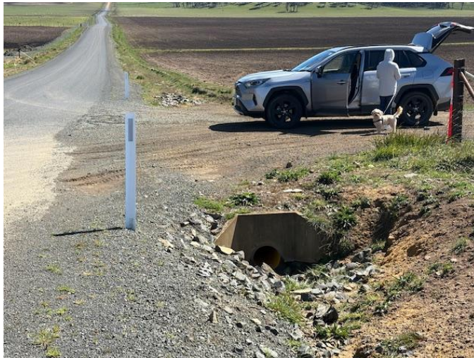
Figure 26 – Farm access culvert inlet
