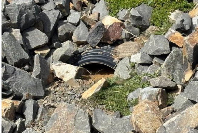
Figure 28 – Farm access culvert outlet
