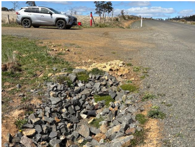
Figure 27 – Farm access culvert outlet
