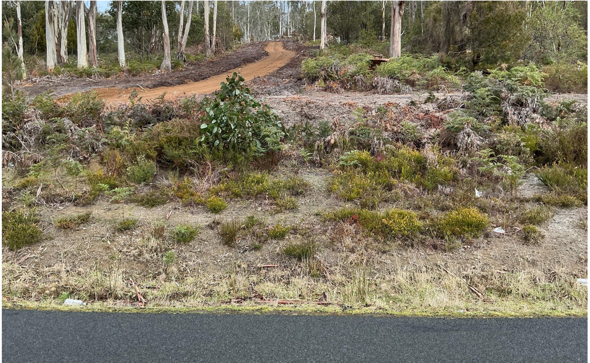
Photo 1 capturing the proposed driveway crossover/cut location which falls within the low landslide hazard overlay
