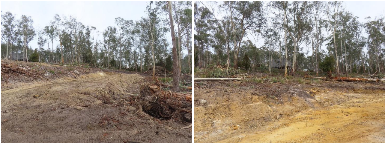
Plates 3 & 4. Views of the existing cleared area
