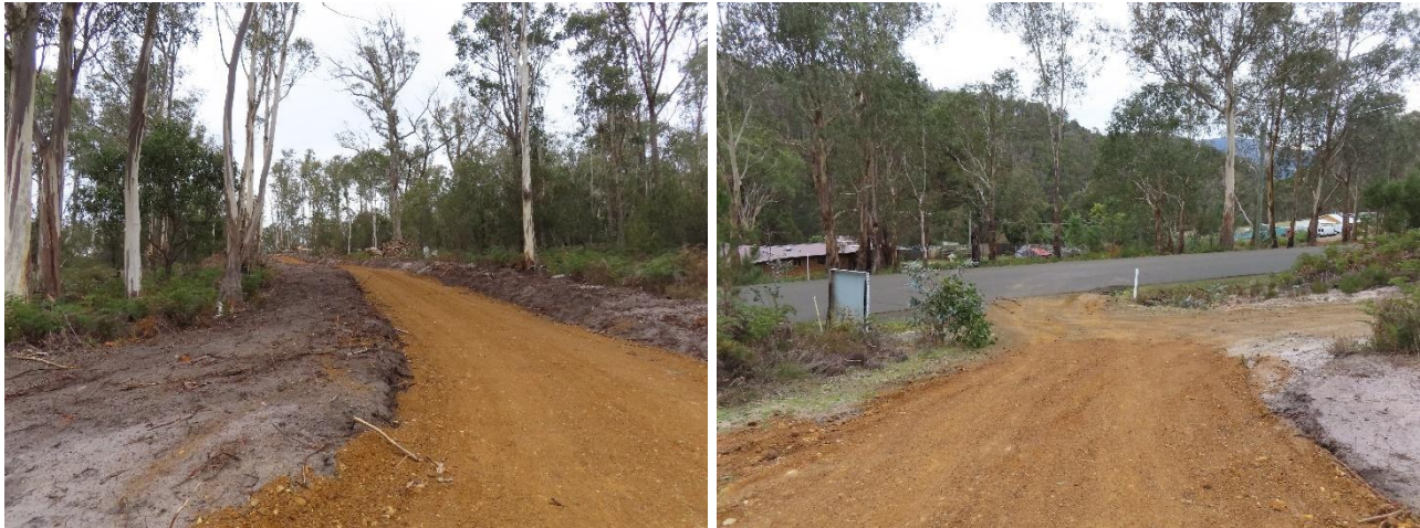
Plates 1 & 2. Views of the existing well-formed access
