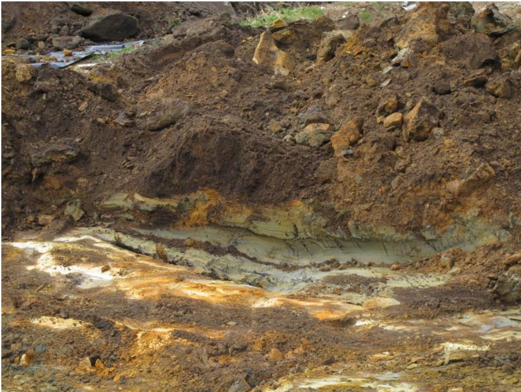
**Figure 3.** Excavations in February 2018 at the site of the former above-ground diesel storage tank (AST) exposed stained, low-permeability clayey subsoil which would have inhibited vertical infiltration of contaminants to groundwater. The diesel penetrated to sandstone bedrock.
