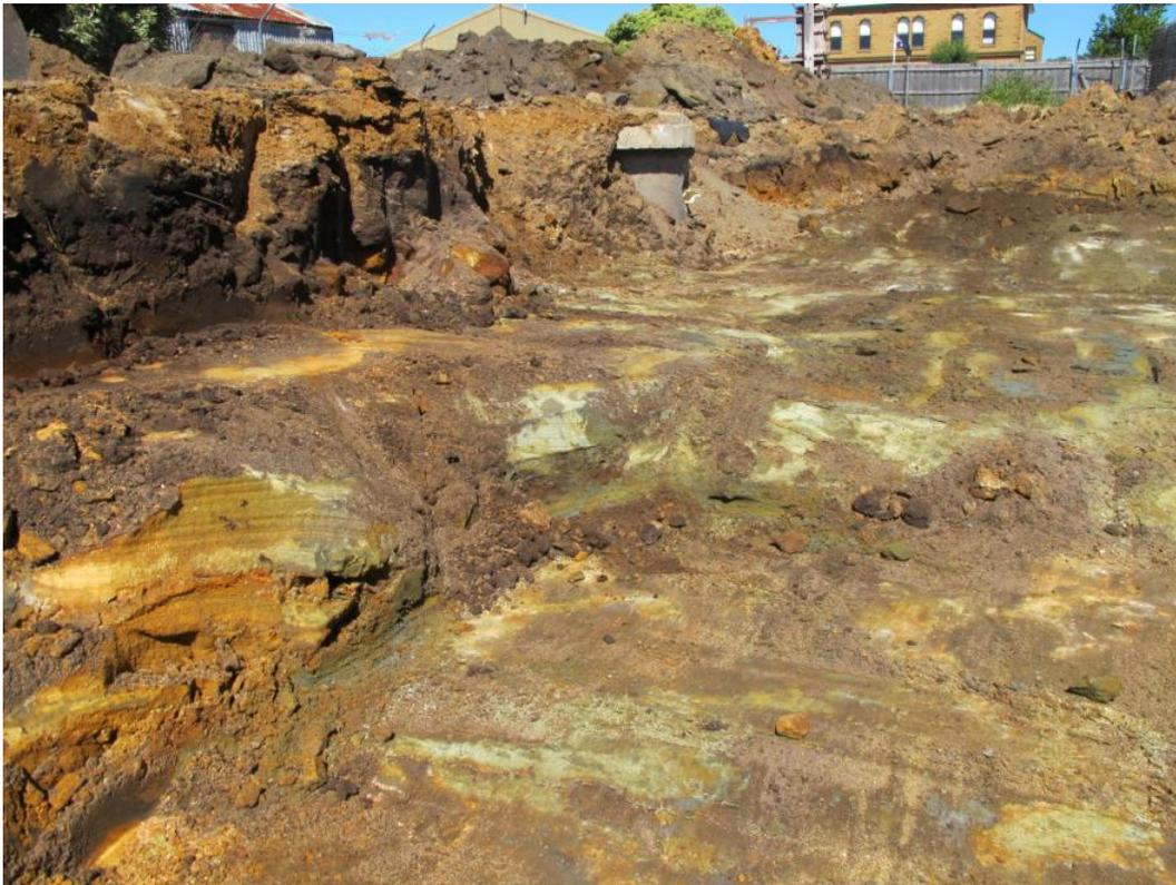
**Figure 3.** Excavations in February 2018 at the site of the former above-ground diesel storage tank (AST). Staining has extended to subhorizontal, clay-filled fractures in bedrock (centre of photo) but the bedrock appears relatively sparsely jointed. There are no apparent steeply-dipping fractures, but if they are present, vertical migration of contaminants is possible but may be inhibited by clay linings.
