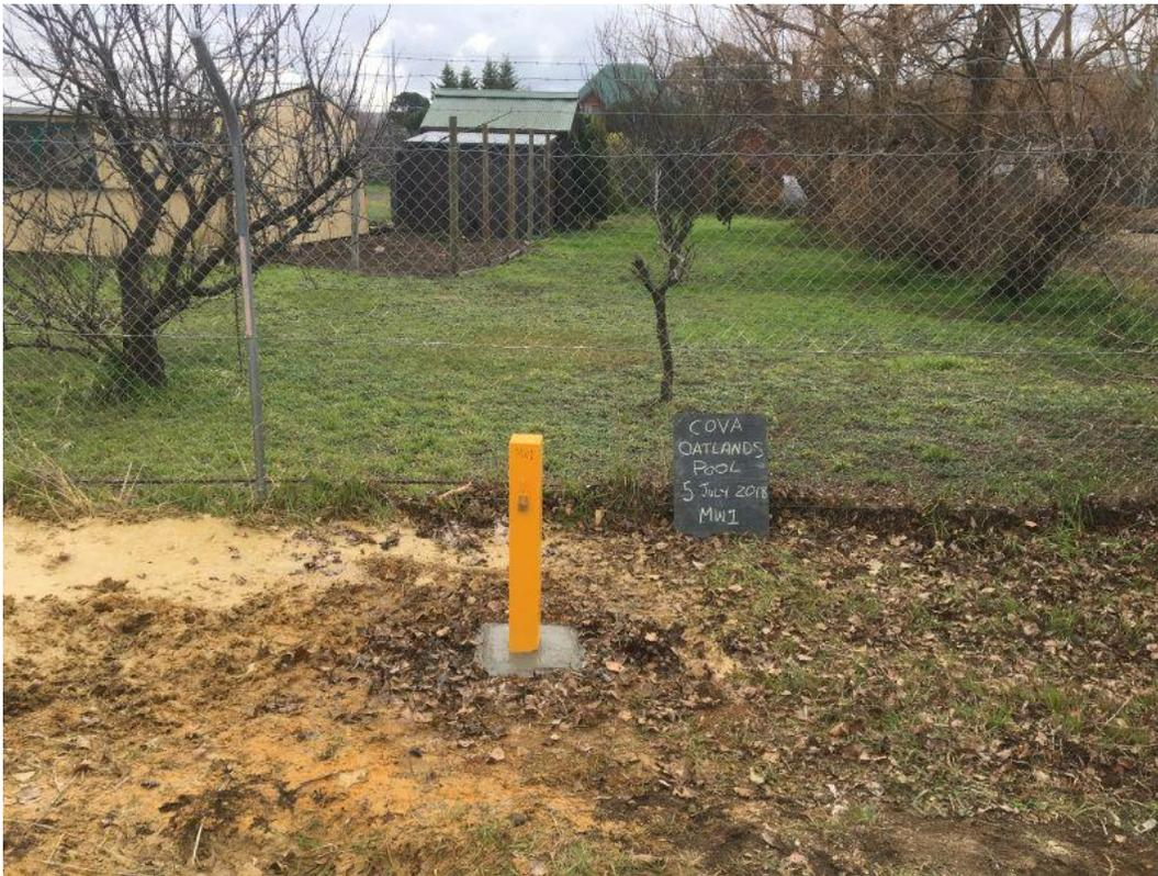
Plate 1.5. MW1 completed with lockable monument, 5 July 2018.
