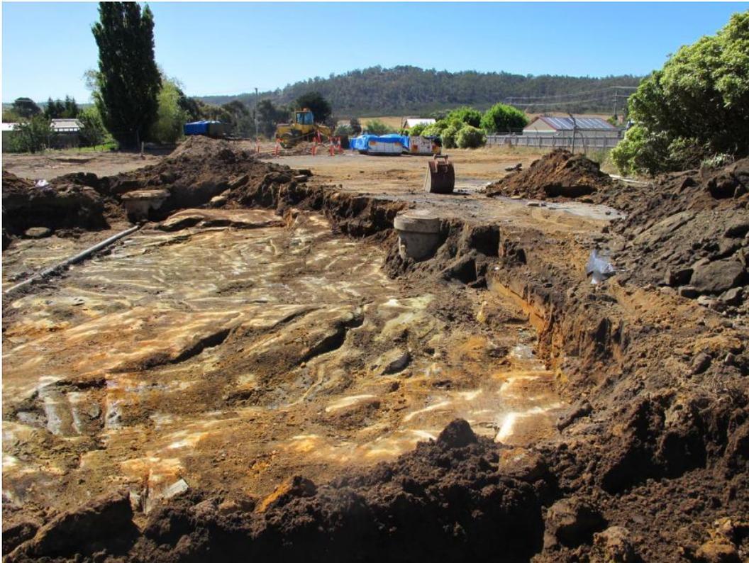
**Figure 1.** Excavations in February 2018 at the Works Depot to remove identified diesel contamination at the site of the former above-ground diesel storage tank (AST).
