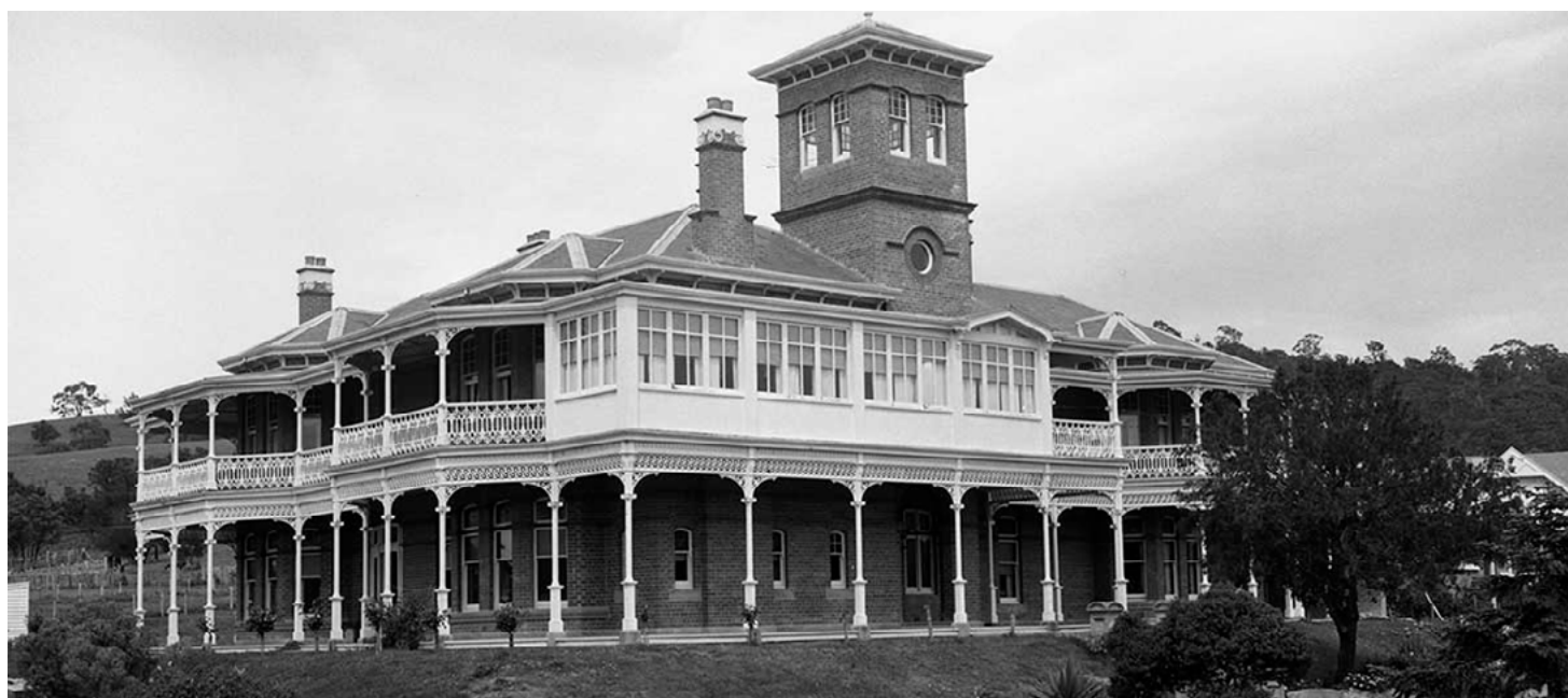
Wybra Hall, Mangalore, built 1900s ourtasmania.com.au
