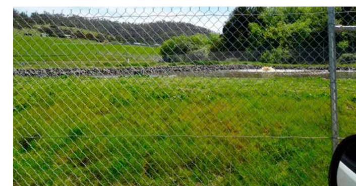
Sewer treatment plant
