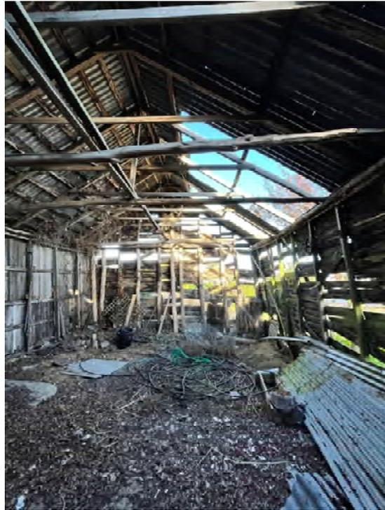
You can see the building as it currently stands. Sheets of roof that fly off in winds are being handed back by neighbours and then stacked in the shed. Majority of timber is completely rotten.
