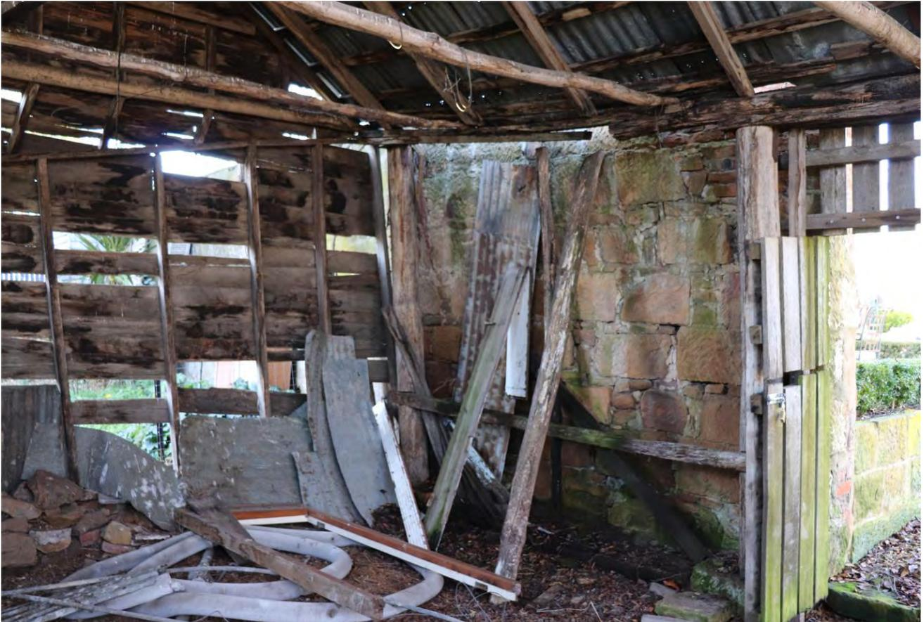
Failed wall framing, lack of base plates and discharge of rainwater onto significant stone wall (to be retained).
