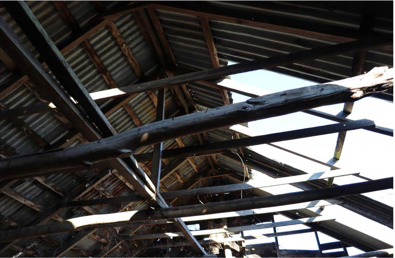
Roof framing in poor condition.
