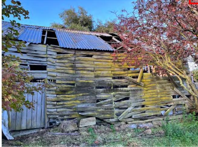
The back exterior of the shed is completely weather worn, rotten and the roof sheets are completely unsafe.
