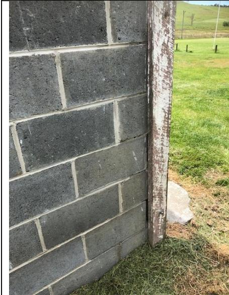
Masonry at the front of the change rooms is being held in place with timber bolted through masonry to timber on the opposite side of the wall. The reason for the cracking to the floors is that the oval side of the change rooms is sinking.
