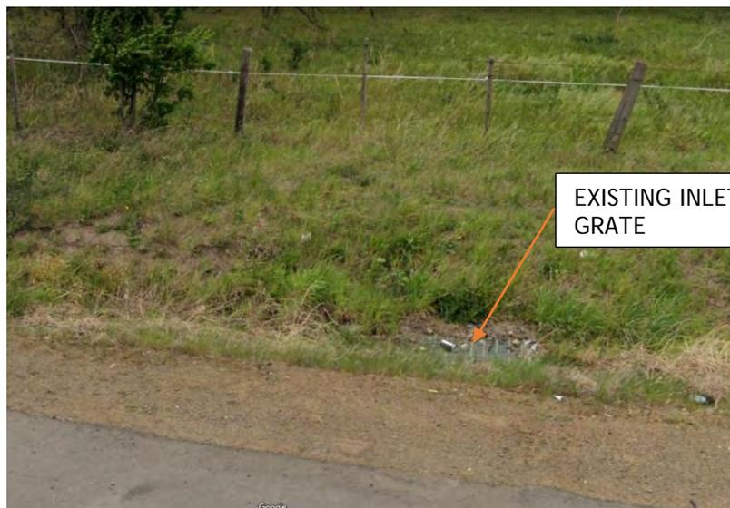
Image 7 - Existing Inlet Pit Midland Highway Table Drain
