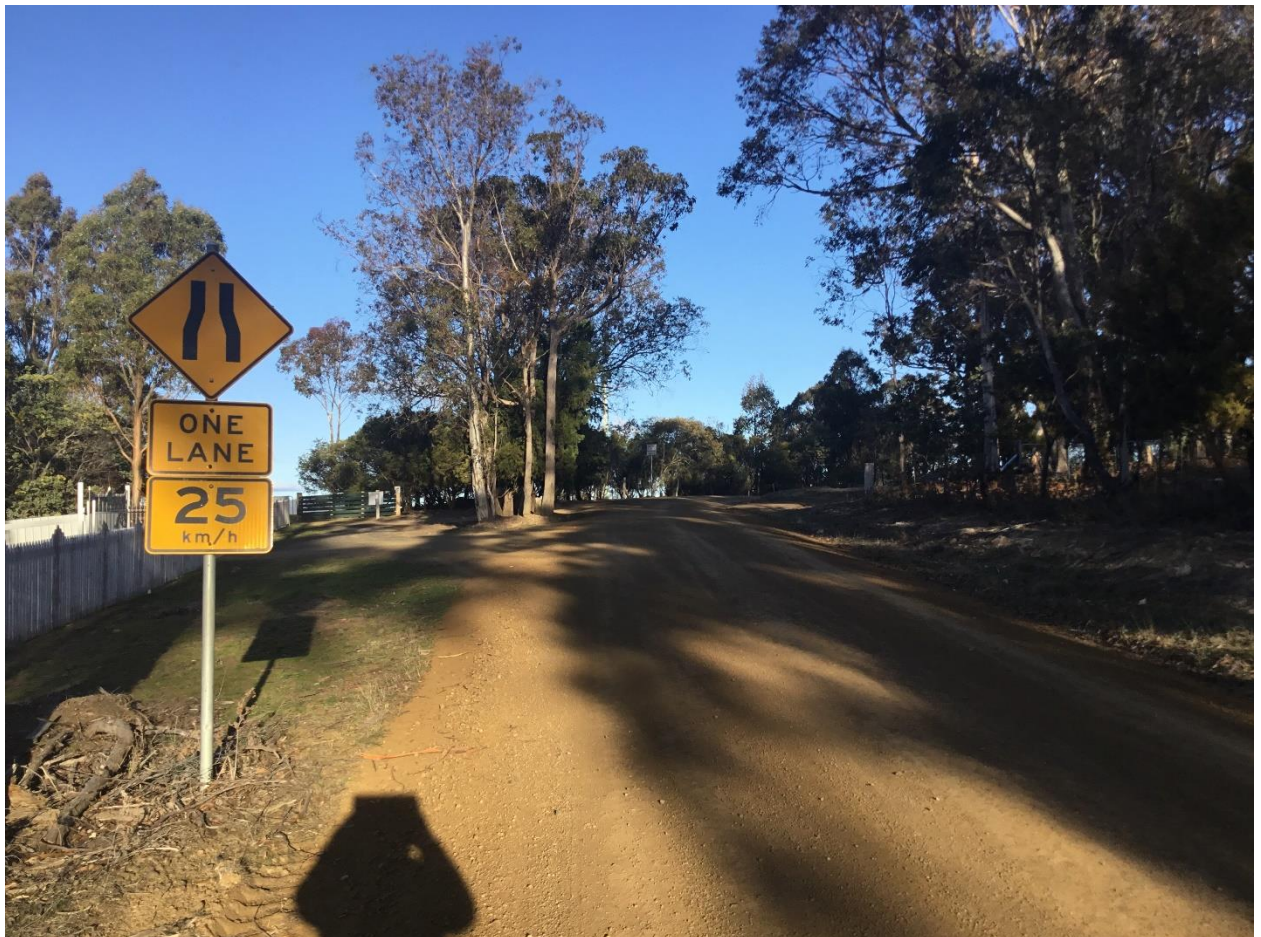
Figure 11 - "Road Narrows - One Lane - 25 km/h" advisory signage on the southbound approach, approximately 100m before the trees.
