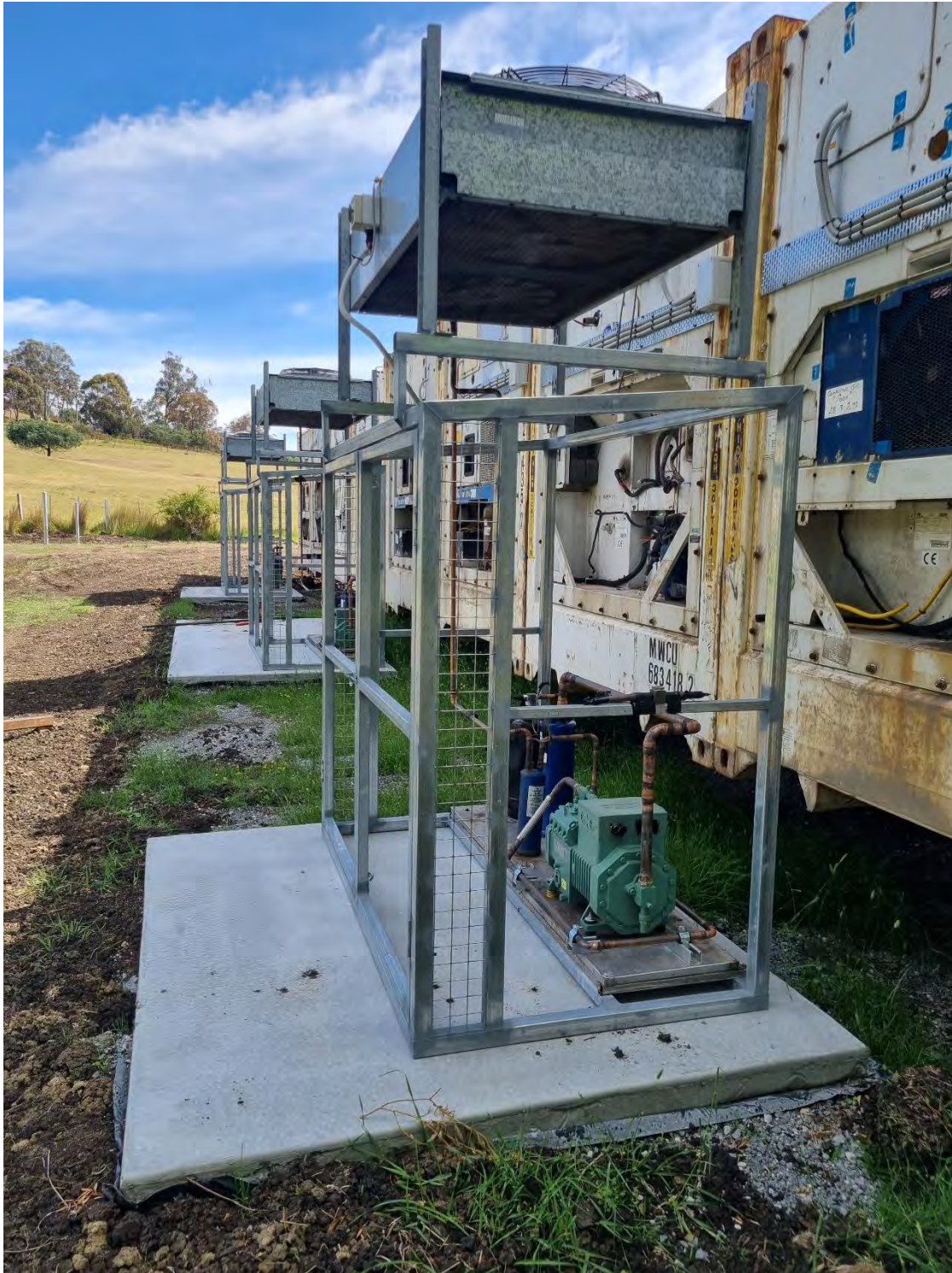
Figure 10: Image showing the three refrigeration units on the western elevation of the Cold Stores, these are yet to be connected.
