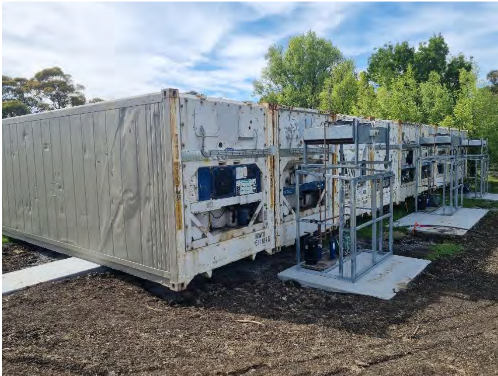
Figure 8: Image of the western elevation of the Cold Stores showing the refrigeration units, which are yet to be connected.
