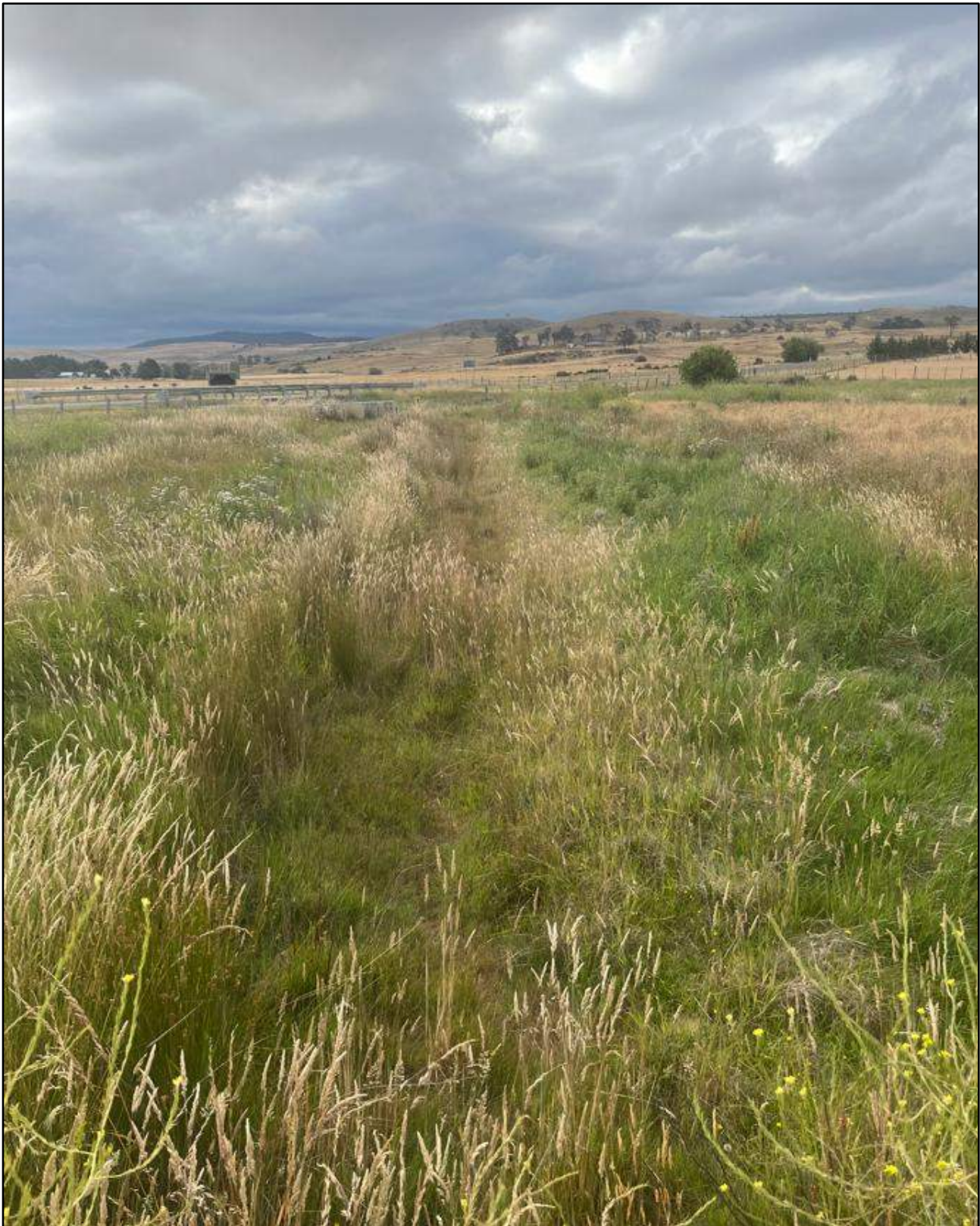
Figure 12. Drain looking north west. Photo: Land Use Planning and Development Tasmania Pty Ltd, taken 14 January 2026.
