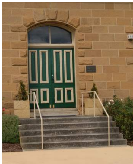
Photo 2 shows the stairway at the main entrance
