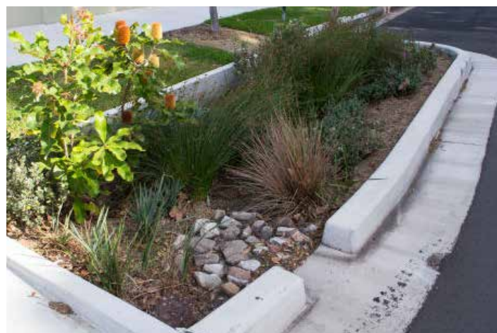
Gaps in kerbs help direct surface runoff into the WSUD gardens.
