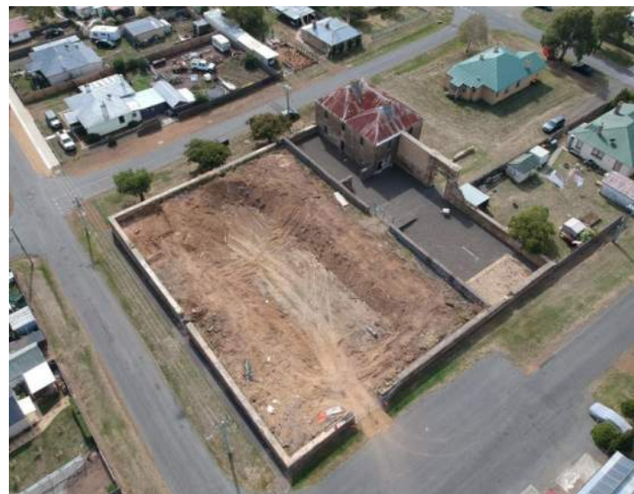
Oatlands Pool during demolition.
