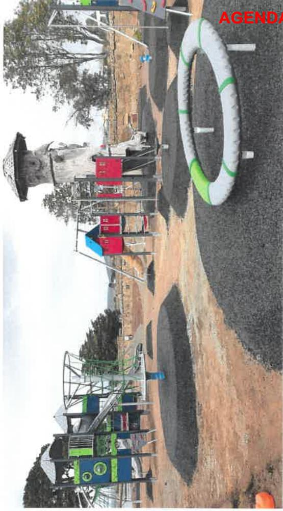
Photo taken 14 September 2020 – getting closer to completion. Final tasks include coating the soft fall rubber, spreading pine bark, finishing the flying fox and installing the last 'spinner'
