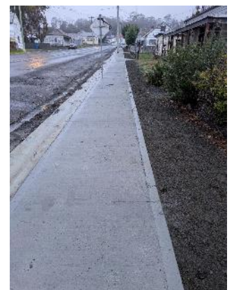
Parattah kerb replacement
