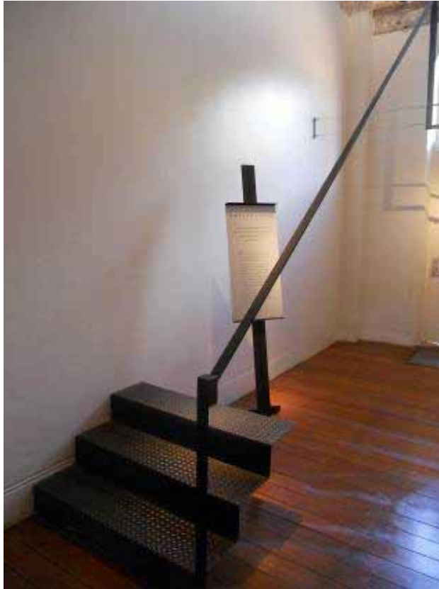
Figure 4.32 – Steel stairs interpreting a former stairway at Hyde Park Barracks, Sydney.
