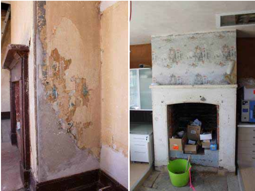
Figure 4.11 (left) – Twelve layers of wallpaper in the Gaoler's bedroom, dating back to 1850. Figure 4.12 (right) – The former women's kitchen, now the artifact lab, where all periods of fabric have been retained, including the 1836 flagstones and fireplace, 1850s plaster, 1930s dado and wallpaper and the 2010 lab fitout. This allows interpretation of 11 phases of history.
