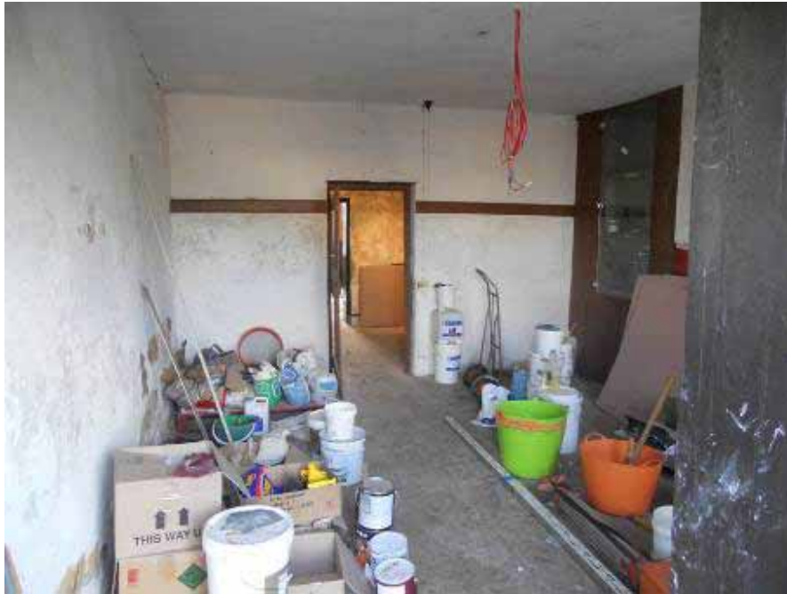
Figure 4.3 - Currently being restored, the former Men’s Kitchen will soon provide 22 square metres of easily accessible public interpretation space.
