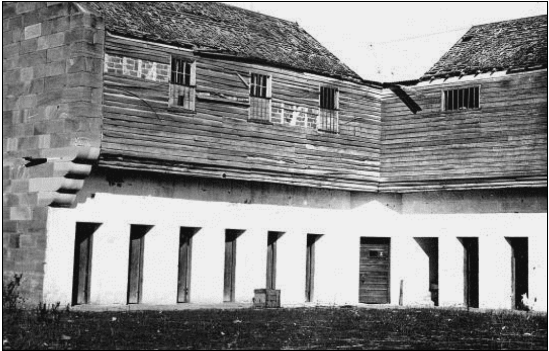
Figure 1.35 – The Men's Division, showing solitary cells with chapel above c1926 (State Library of Victoria Heritage Collections).
