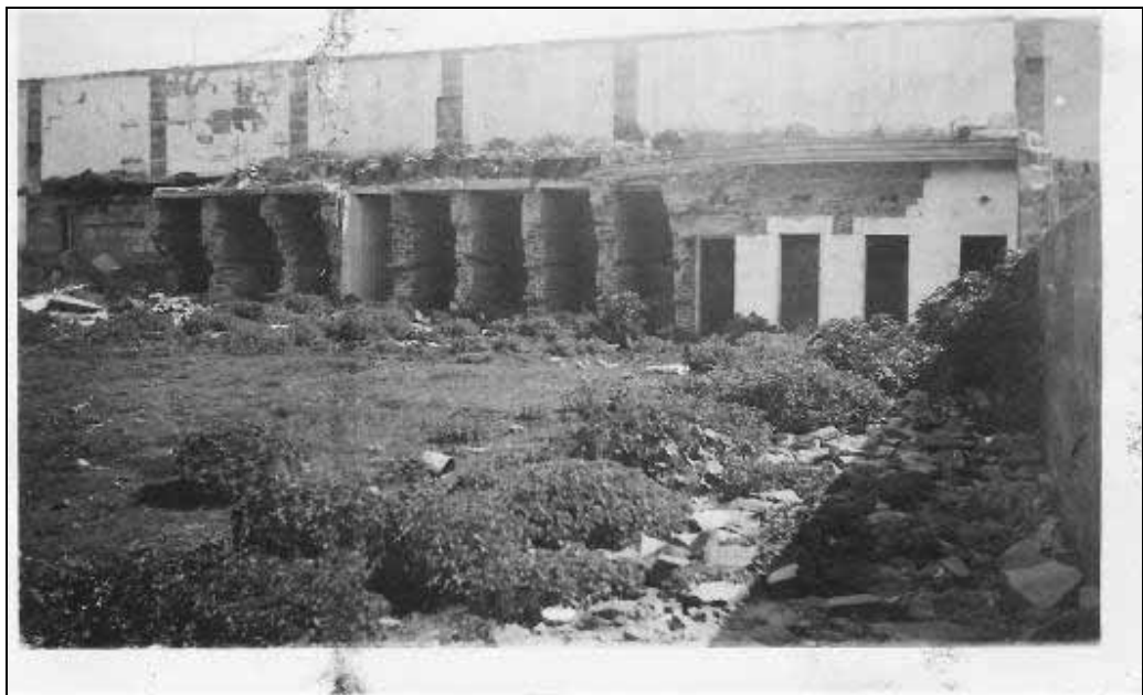
Figure 1.41 – Demolition of the Men's Division, late 1937 (photograph loaned by the Oatlands District Historical Society).
