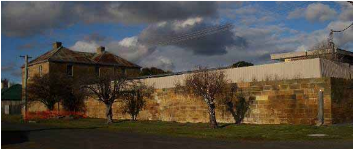
Figure 1.1 – Western wall of the Oatlands Gaol
