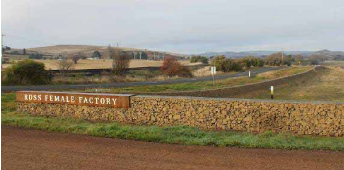
Figure 4.27 – Gabion walls at the Ross Female Factory.
