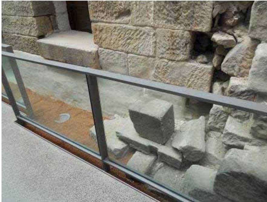
Figure 4.34 – Jagged wall edges at the Sydney Mint, showing where building elements have been removed.
