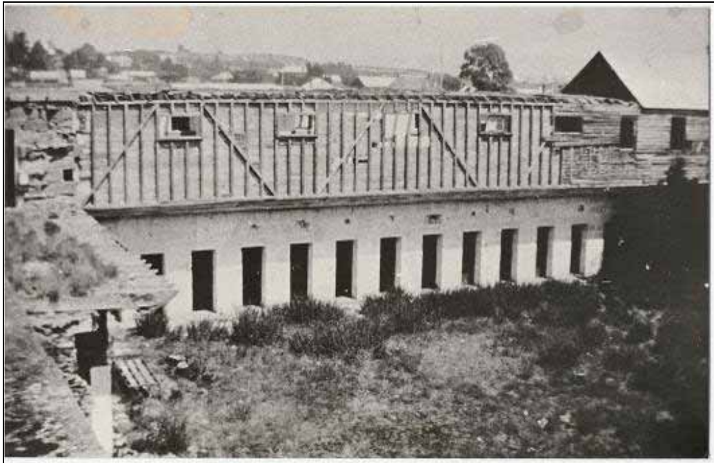
Figure 1.40 – Demolition of the Men's Division, late 1937 (photograph loaned by Graeme Raphael, Oatlands).
