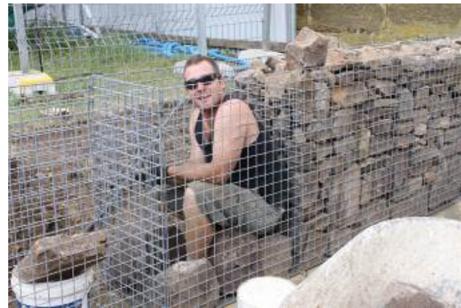
Matt Rooke of Rock on Rock Garden Escapes works on gabion stone walls at the Oatlands Gaol. Photo – Brad Williams
